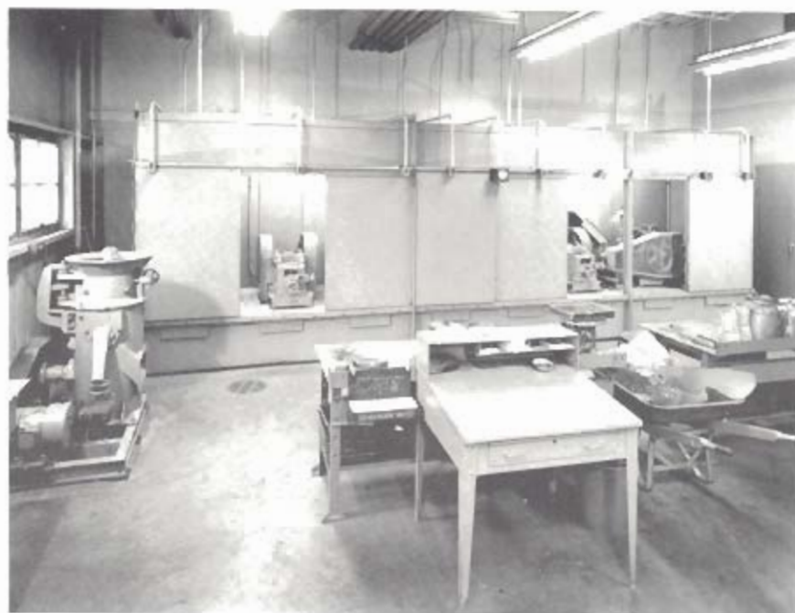
Pulverizing machinery is enclosed in a dustproof cabinet to minimize the possibility of sample contamination and provide for better housekeeping.
